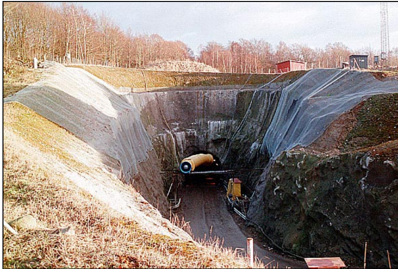
Figure 5. The working tunnel on the Hallandsås ridge. Photo: H-G Wallentinus, January 2000
