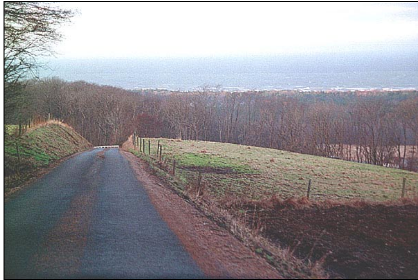
Figure 3. The slope of the Hallandsås ridge towards the north-west. The northern tunnel mouth is situated to the right of the photo. Photo: H-G Wallentinus, January 2000
