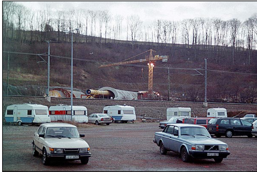
Figure 4. The northern tunnel mouth. Photo: H-G Wallentinus, January 2000
