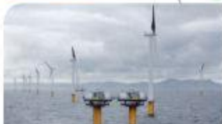
Robin Rigg windfarm
