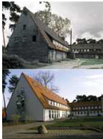
Former military horse stables in Potsdam, Germany, have been converted into an office building.
