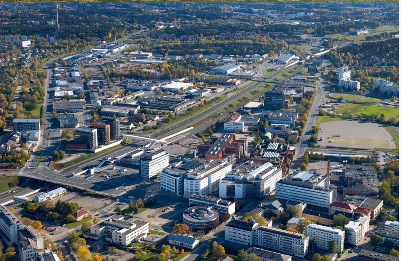
The Itäharju area was chosen as Turku's pilot site in the Baltic Urban Lab project Photo: Suomen Ilmakuva Oy
